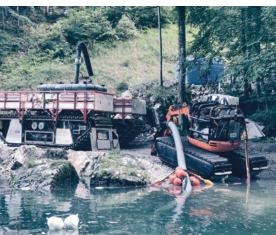
To restore the La Balme-de-Rencurel reservoir, whose access is highly constrained by a narrow road and a steep track at the tail end of the reservoir, Watertracks deployed the NESSIE® underwater robot for the main dredging operation. Sediment discharge was carried out in a controlled manner immediately downstream over the dam crest.
